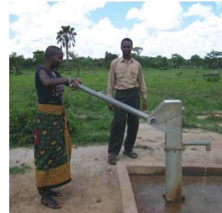
The borehole at Mwanhala village
